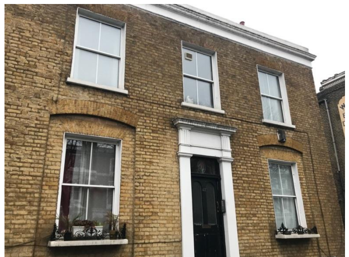
Figure 12 No. 47 Trafalgar Avenue
