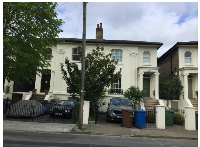
Figure 4 Nos 30, 32, 34 Glengall Road
