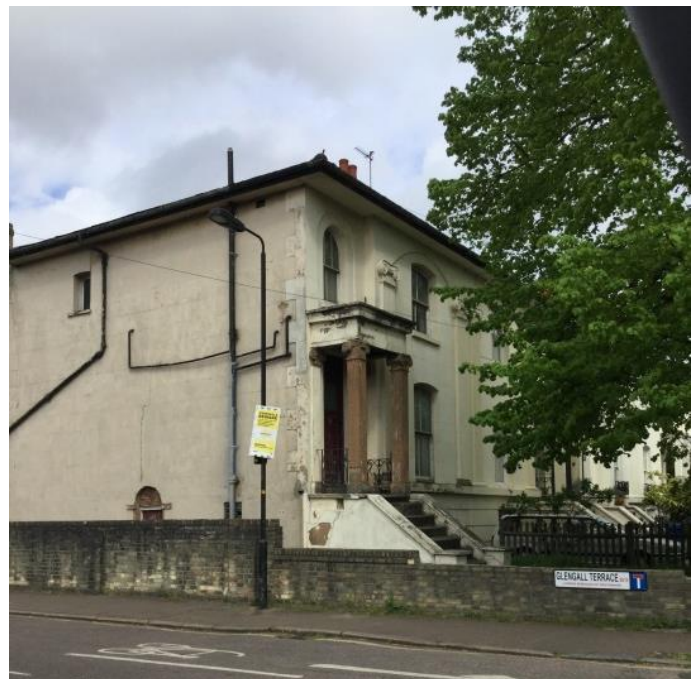
Figure 9 No. 38 Glengall Road
