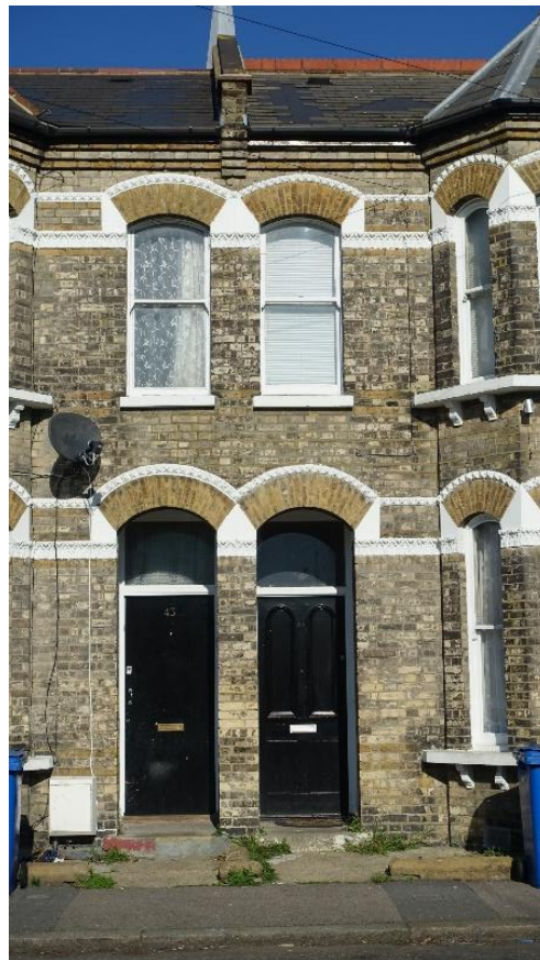
Figure 15 Late Victorian terraced houses: Loncroft Road (detail)
