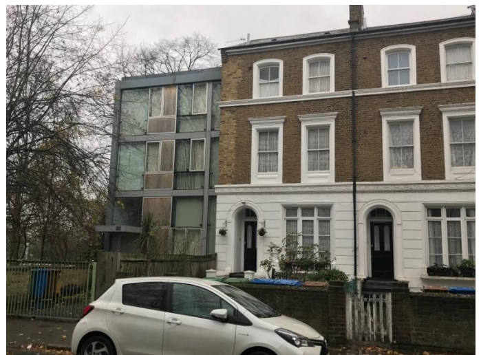
Figure 11 No. 66 Trafalgar Avenue
