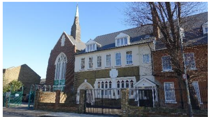
Figure 7 Peckham Mosque with former hall and rectory
