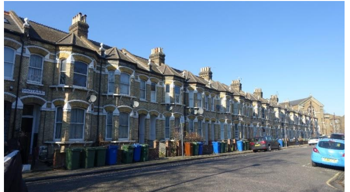
Figure 14 Late Victorian terraced houses: Oakley Place
