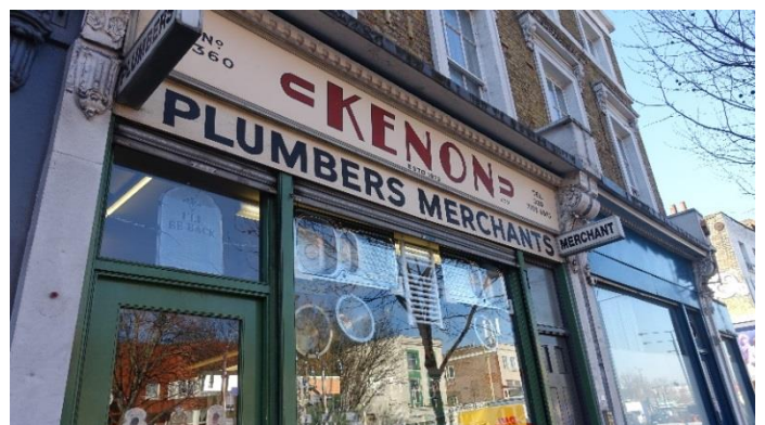
Figure 20 Shopfront detail: No. 360 Old Kent Road
