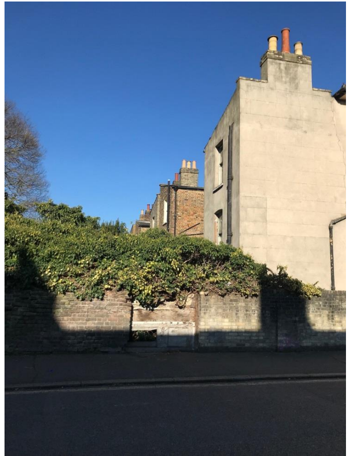
Figure 4 Rear elevations Nos 34, 36, 38 Glengall Terrace
