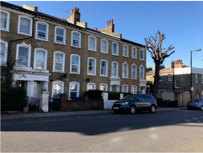
Figure 6 Nos 40–46 Glengall Road
